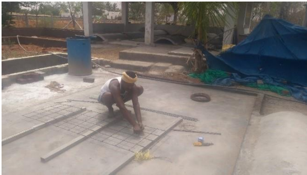
1. Steel rods base for slab making
