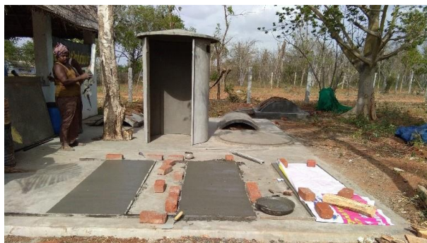
5. Slab curing for doors
