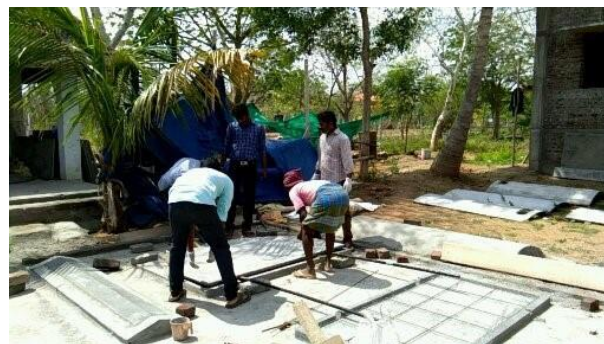
6. Joining slab mould and doors at platform
