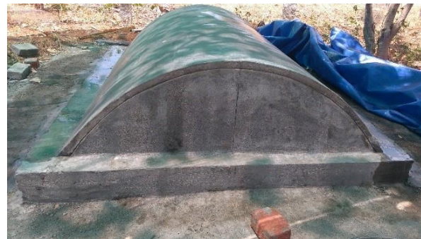
4. Base Mould for fabricating circular slabs
