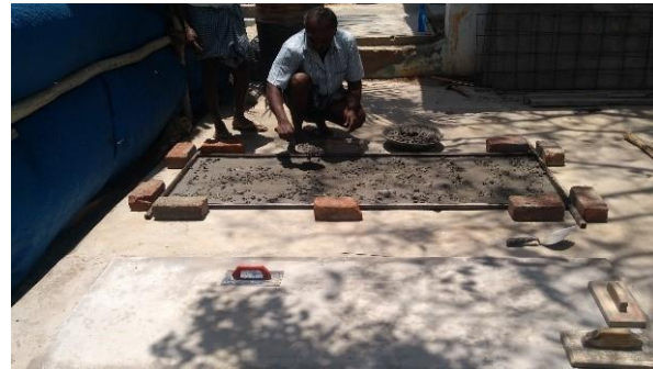
2. Applying cement and sand mixture
